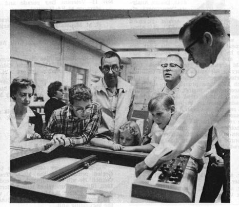
PLOTTER BOARD of Sandia's analog computer and Ken Bixler (9411), right, show visitors how computers solve problems. The graph reflects trajectory of rocket launch, orbit, and reentry.
